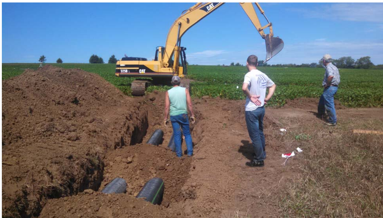
Figure 3. Installation of pipe outlets (Aug. 29, 2014).
