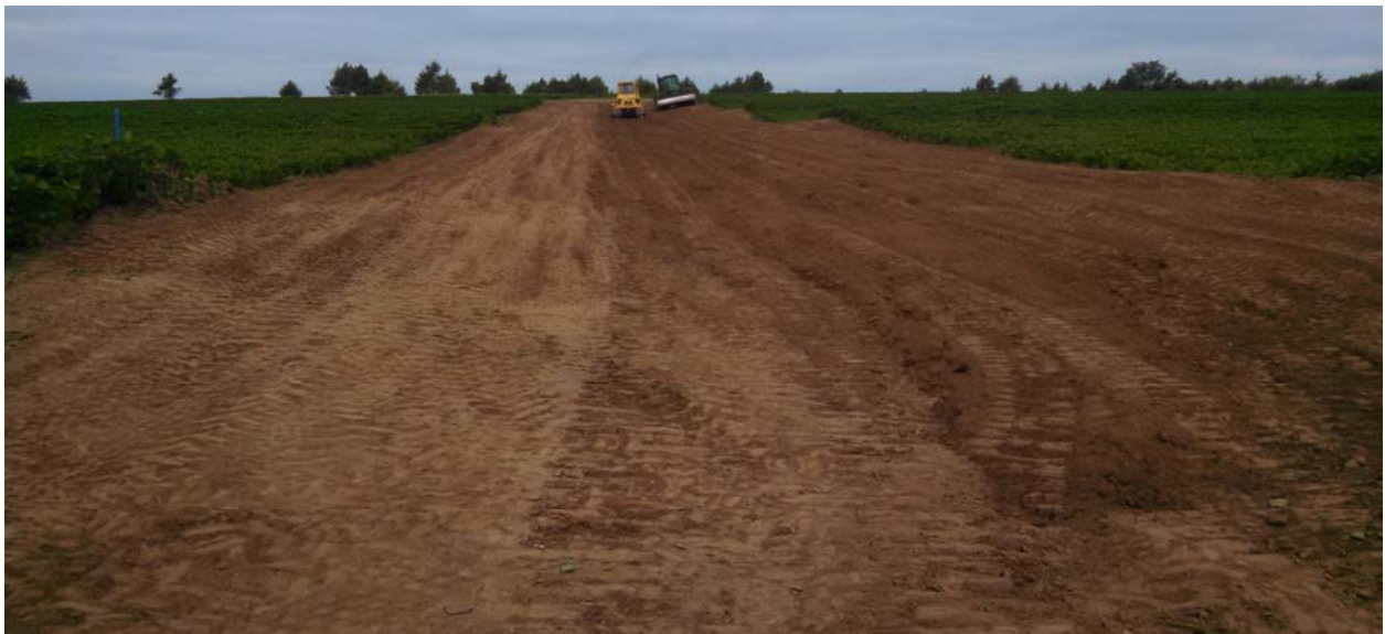
Figure 2. Waterway construction (July 18, 2014).
